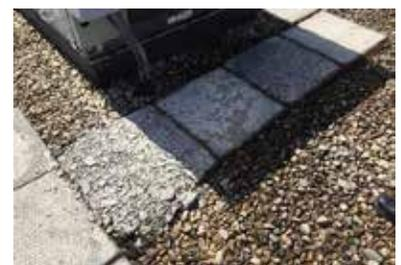
more years whereupon it should be replaced. A non-ballasted system is recommended with a light-colored membrane with a long warranty.
