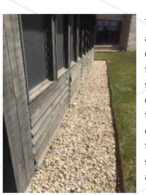
The porches provided on the west and east sides of the building have cedar siding and a cedar-trimmed fascia. This has weathered and has started cupping, with nails sticking out. The boards should be re-
